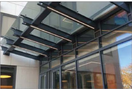
Entry Canopy Lighting Linear luminaires integrated with the main entry canopy structure invites pedestrians in.
